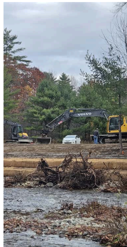
Root wads & erosion repair in Orford, NH (before the buffer planting).
